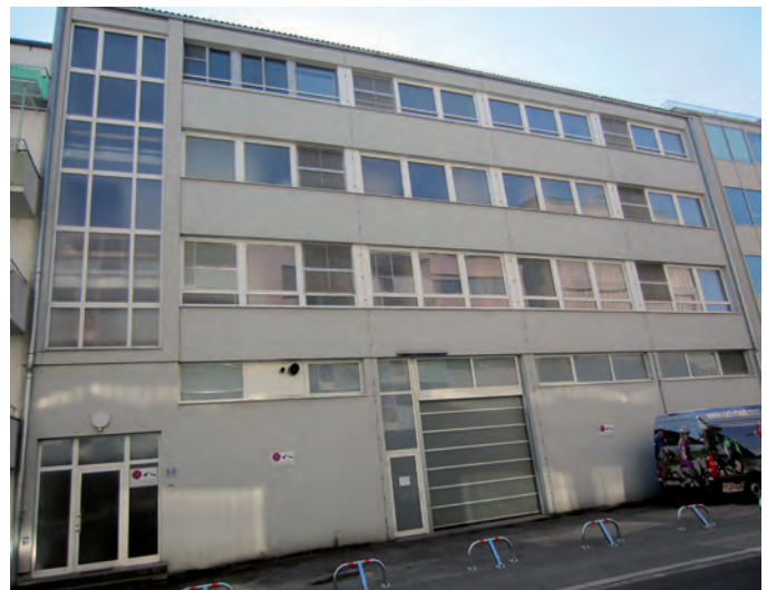
Fig. 6: Depository "Lindengasse" is named after the street where it is situated. At special occasions guided tours show the usually hidden background.
