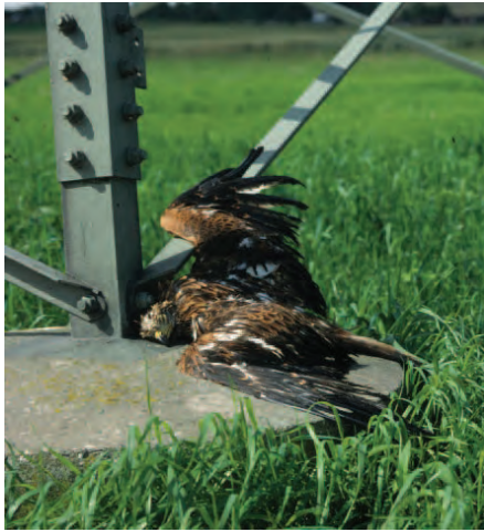
Toter Rotmilan am Mast (Foto: Archiv VSW)
