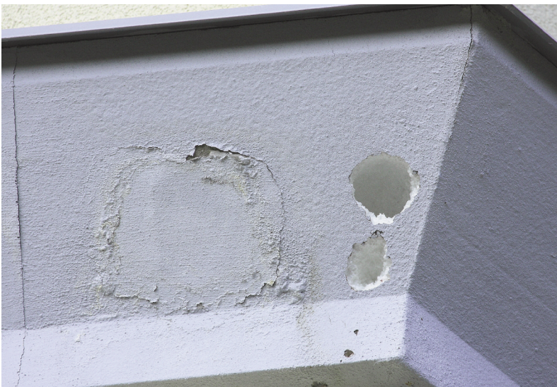
Fig. 14: Start cavity in a styrofoam insulation. Photo: Z. Orban.
