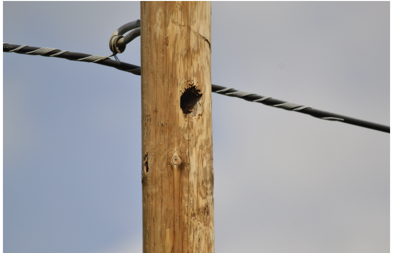
Fig. 1: Woodpecker cavity in a utility pole. Photo: G. Gorman.
