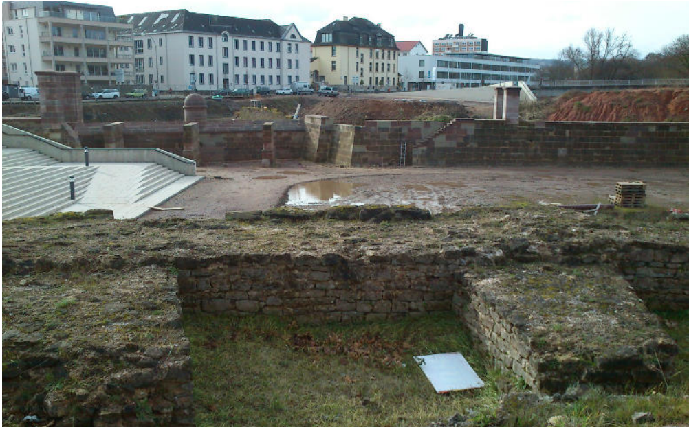
Abb. 6: Baustelle am Ravelin V.
