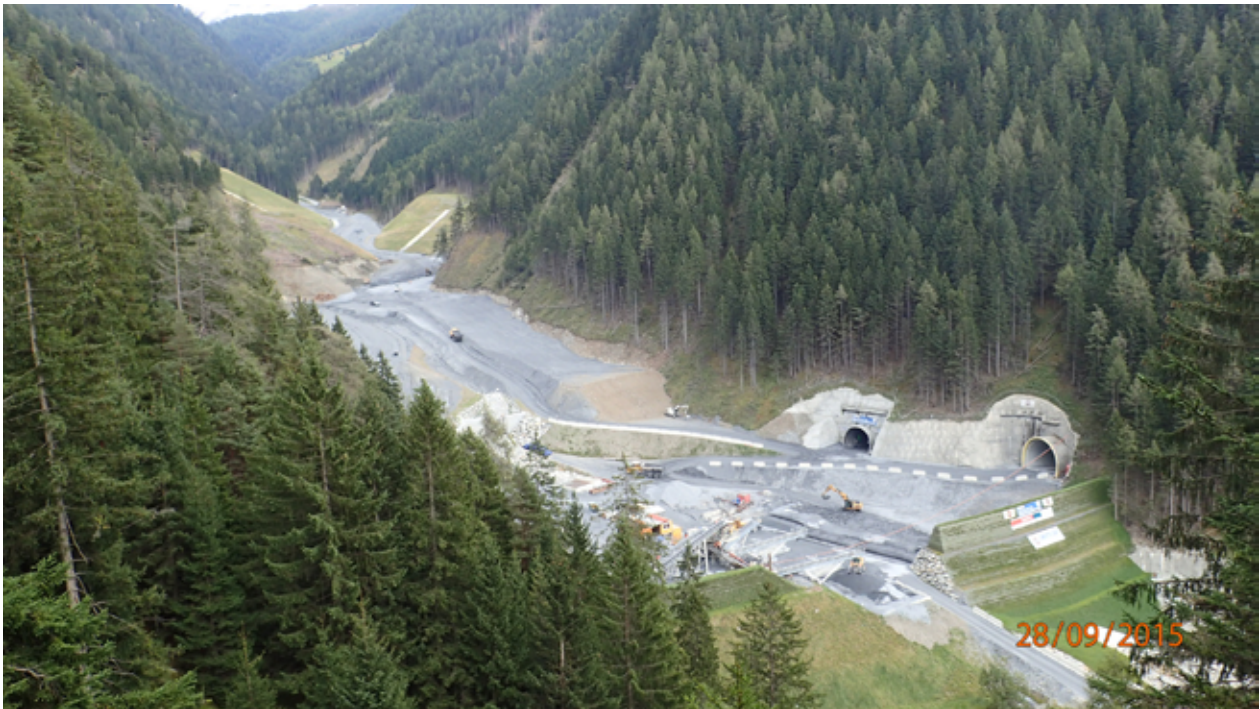
Fig. 5: Overview of the Padaster valley (Status 09/2015): the depositing of excavated material in the main disposal phase is in progress.
