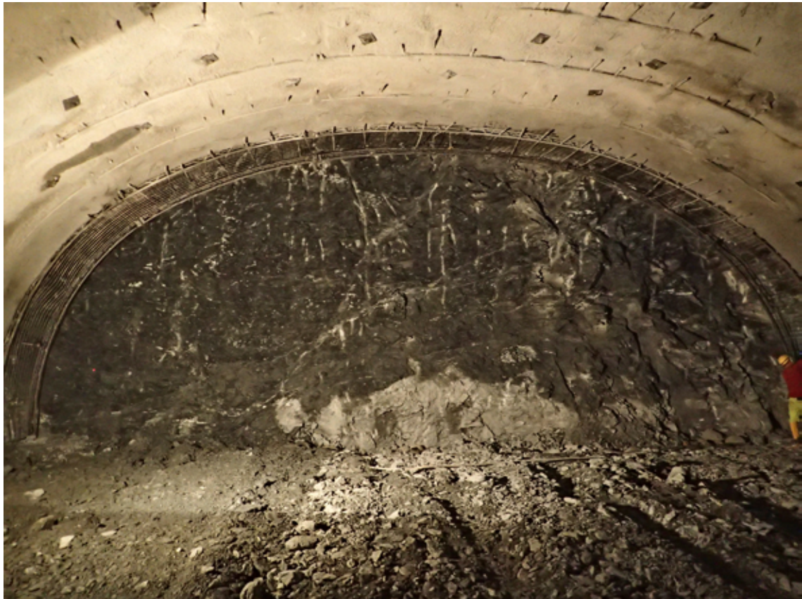
Fig. 11: Tunnel face of the connecting tunnel: quartz phyllite.
