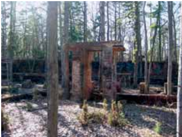
Abbildung 2: Brooksbrae Brick Factory, Manchester Township, NJ (Foto: Cha-Wen Rung)
