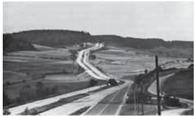
Visually disjoint arcs and tangents (above) versus a continuous, smoothed ribbon (below).
