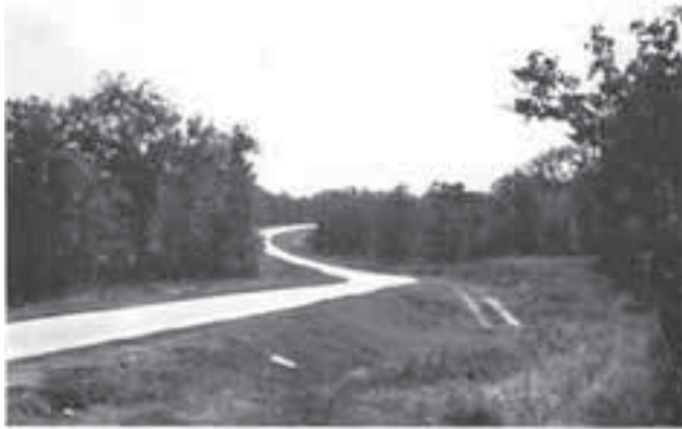
SHARP TURNED CURVES ON AN OLD-TYPE HIGHWAY
