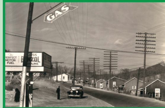
Roadside Gas Station with Miner's Houses across Street, Lewisburg, Alabama, December 17, 1935 © Walker Evans Archive, The Metropolitan Museum of Art
