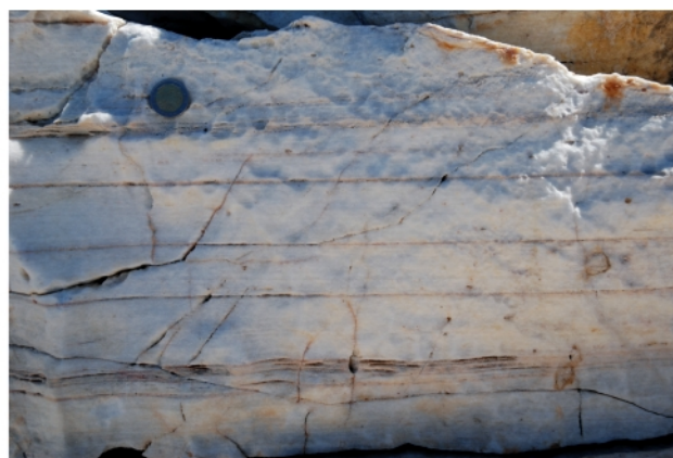
FIGURE 7: Comparison between building stones with outcrop lithologies on Despotiko. a) Two building stones from Building A consisting of marble 1 (centre and left part) from the east façade of room A1. Note the carefully dressed surfaces, the white, slightly greyish colour and especially the characteristic rose-coloured layers of fine grained dolomite marble. The building stones below and to the right comprise white mylonitic gneiss. b) Outcrop photograph of marble from Cape Koutsouros (for location see Figure 3), comprising white, medium grained calcite marble with well developed foliation and characteristic rose coloured, thin dolomite marble layers. Note the close similarity with marble 1 from Building A (for colours see the online version of this paper).
