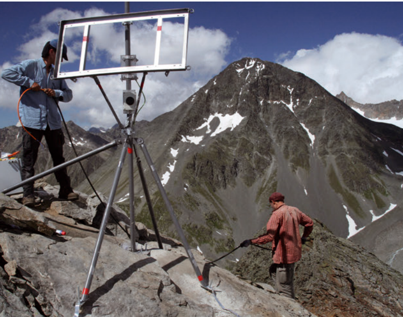
Fig. 5: Installation of an automatic snow camera at 3 100 m.
