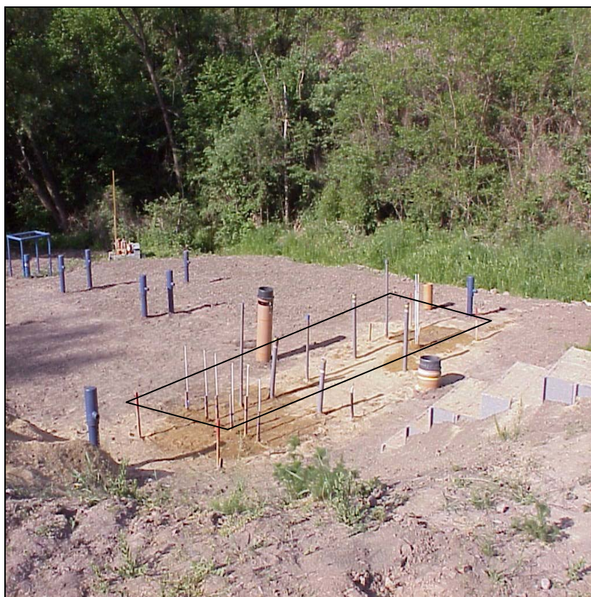
Fig. 14: Position of PRB with monitoring wells
