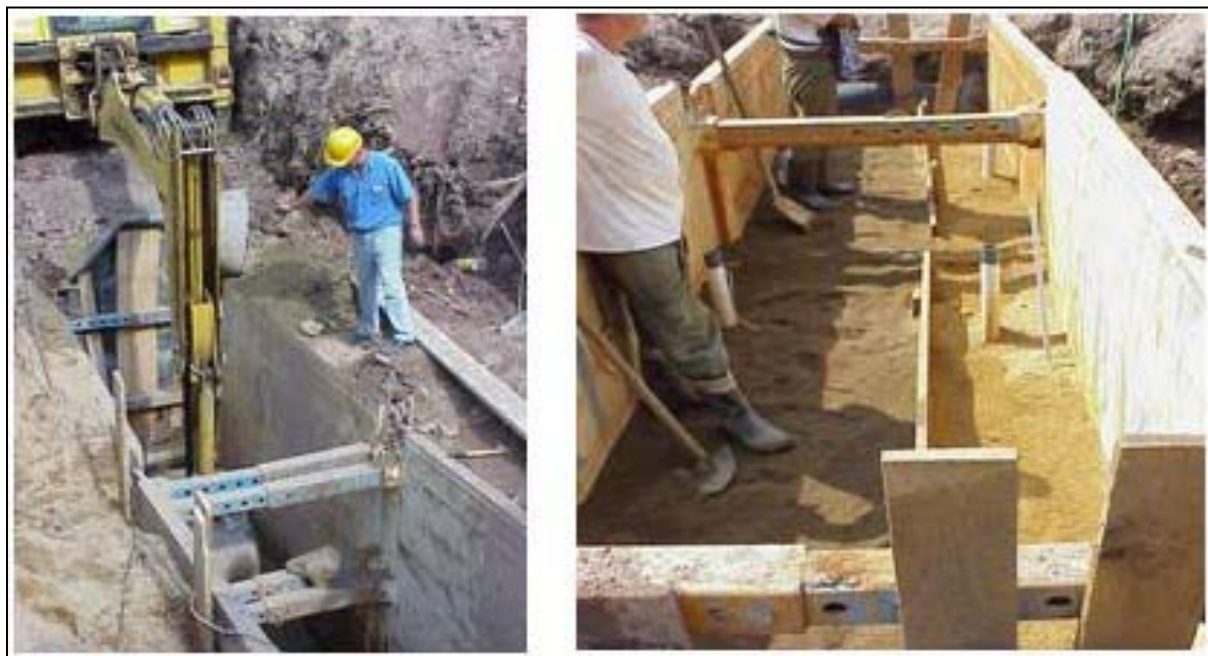
Fig. 13: Construction of the experimental PRB in Zsid valley near Pécs.
