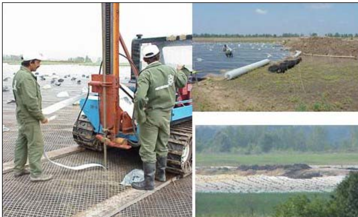
Fig. 11: Covering of soft tailings using geomaterial and vertical drains.
