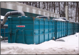
Containerbiofilter
