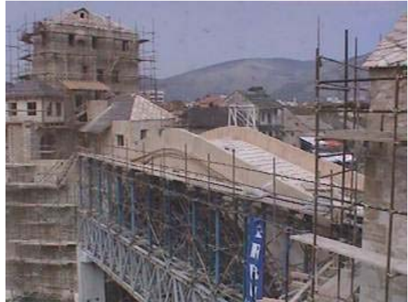
Fig. 2. The bridge under reconstruction
