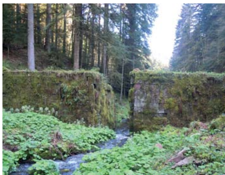
Abb. 7: Bergseite hintere Lay-Schwallung. Fig. 7: Mountain-facing side of splash dam Hintere Lay
