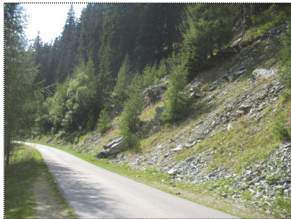
Text-Fig. 4.10: Left: The potential rockfall hazard along the Asten Road, caused by the sagging slope within the deformation near Moharspitz. Right: Rockfall boulders close to houses on the upper slope of the sturzstrom Moharspitz towards the Moell Valley. (Source: S. MELZNER, photographic archive of the Geological Survey of Austria).
