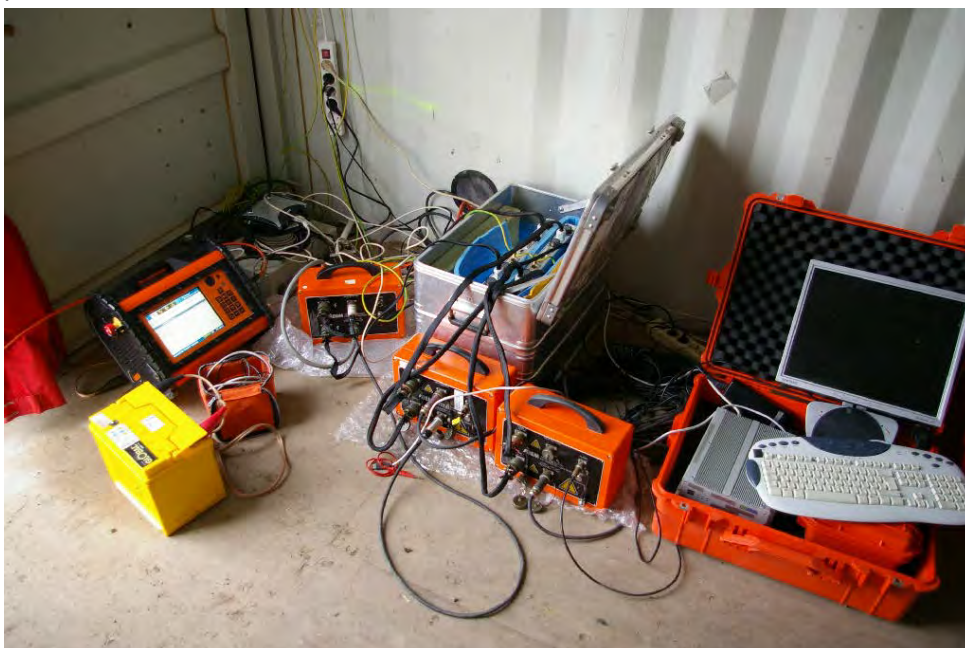
Fig. 3: Temporary installation of the present data acquisition system on a landfill in 2011.
