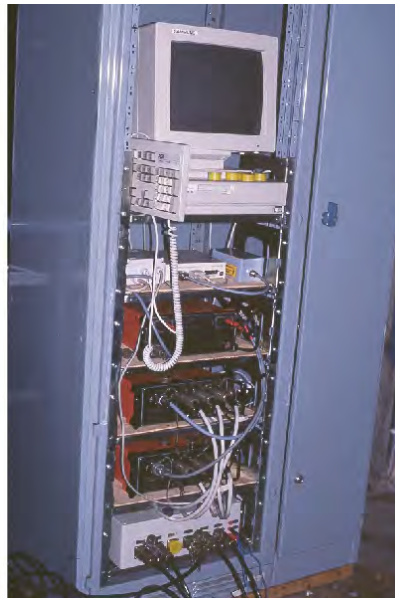
Fig. 2: The first permanently installed data acquisition system on Hällby embankment dam, installed in 1996.
