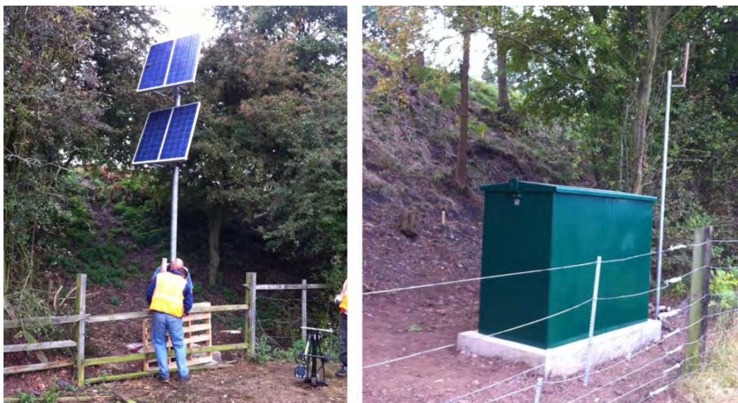
Fig. 3: Installation of ALERT monitoring instrumentation at the GCR(N) test site.
