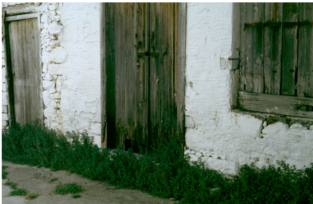
Fig. 4: Parietaria judaica on wall feet in ancient villages.
