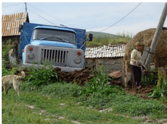
Fig. 72: Manual preparation of dung bricks in Tabatskuri.
