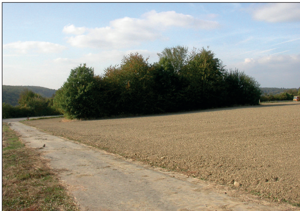
Abb. 6: Bunker 627 (E1) (Foto: Martin Lillig)
