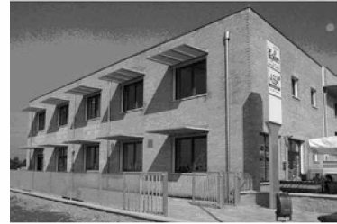
Figure 10: Passive office complex in Santa Croce near Pisa (Gantioler 2008).
