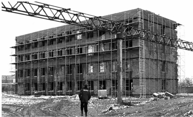
Figure 8: Passive house Moscow Ratmirovo: construction photo (see contribution by [Elokhov]).
