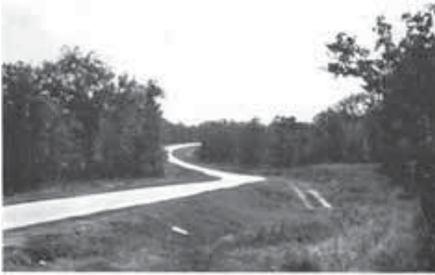
SHARP TURNED CURVES ON AN OLD-TYPE HIGHWAY
