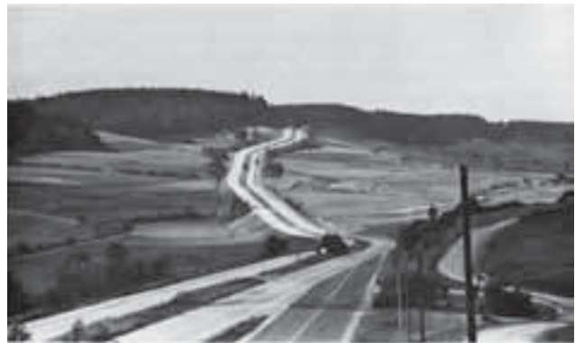
Visually disrupted axis and tangents (above) versus a continuous, smoothed ribbon (below).
