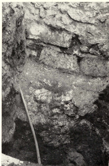
Abb. 16 Fundament, Pfeiler I (k)
