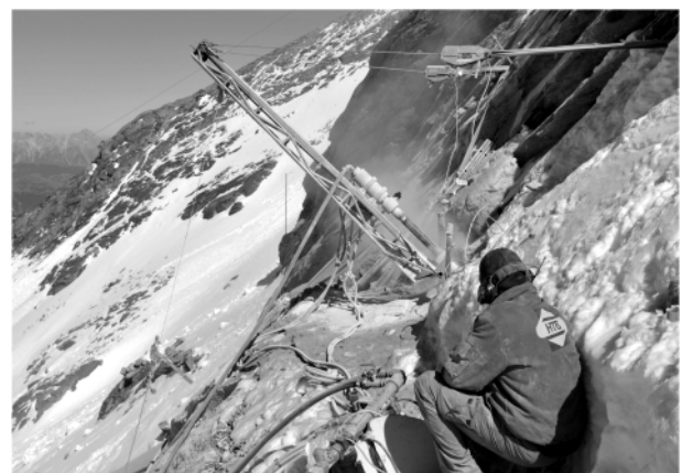
FIGURE 5: Air flush rotary drilling at the Kitzsteinhorn west face in September 2010 (borehole depth 30 m) (Photograph by Ingo Hartmeyer).
