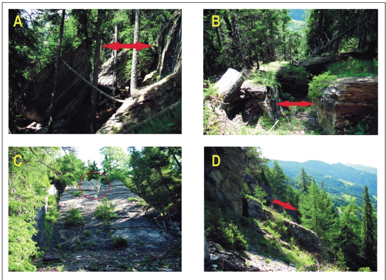
FIGURE 4: Rockslide in micamarble of the Glockner Nappe System (Penninic Unit). (A) The rockslide (GMM 4 in Fig. 1) shows in the scarp area a displacement of about 20 m and highly loosened zones/caves in the upper part (B) Tension fissures strike slopeward following the main fault directions (317/80) (C) Overturning or folding of rock masses at the toe of the slide; possibly rockfall source (red circle) and topple areas (D) detachment of large rock masses by sliding mechanism (photos by S. Melzner, 2010).
