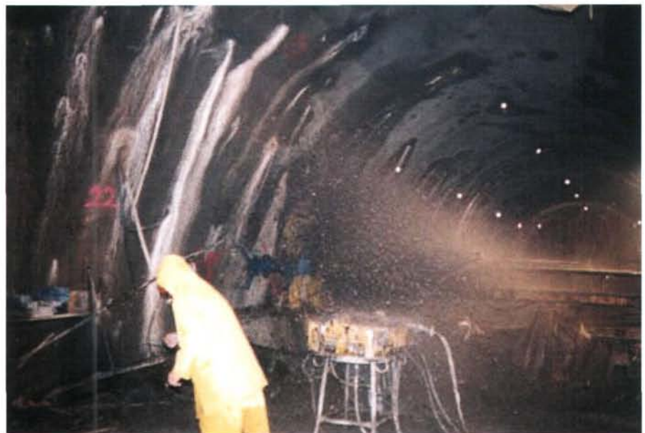
Fig. 9 A dramatic ingress of water (upper photograph) and sand- to gravel-sized dolomitic material (lower photograph), occurred after the drilling of anchor boreholes tapped a cohesionless water saturated fault zone at km 31.23, Brixlegg-East Reconnaissance Tunnel.
