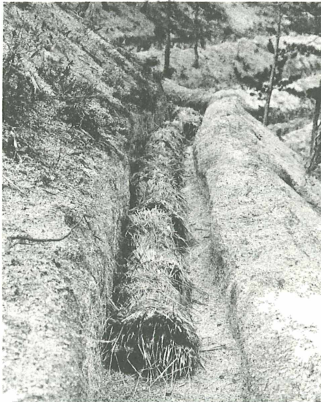
Fig.14 Under execution of the Tending Work B in the declining forest. Straw is put into the excavated trench.
