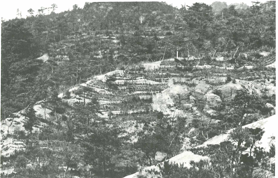
Fig.12 Just after execution of the anti-erosion plantation.
