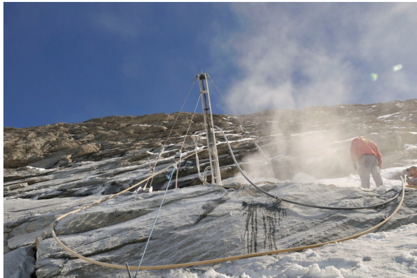
Figure 2: Air flush rotary drilling at the Kitzsteinhorn west face (© Ingo Hartmeyer)
