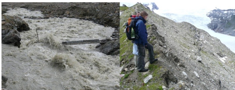
Figure 1: Examples of changes along trails in already ice free areas: Extreme runoff peak of a glacial stream flooding a bridge in ÖtztalerAlpen (left). Partial destruction of a trail along the ridge of the 1850-moraine along a glacier in Venedigergruppe (right). © Erich Heuke
