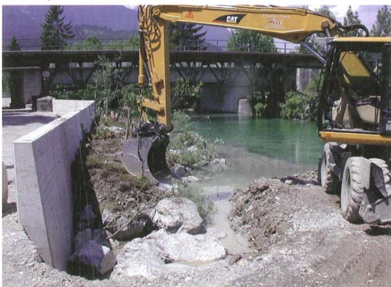
Fig. 5: Necessary engineering measures for flood protection were implemented in the Archbach considering habitat requirements of the indigenous stone crayfish. Today these rocks with some vegetation cover provide a complex habitat for the highly threatened crayfish A. torrentium (Foto: L. Füreder).
