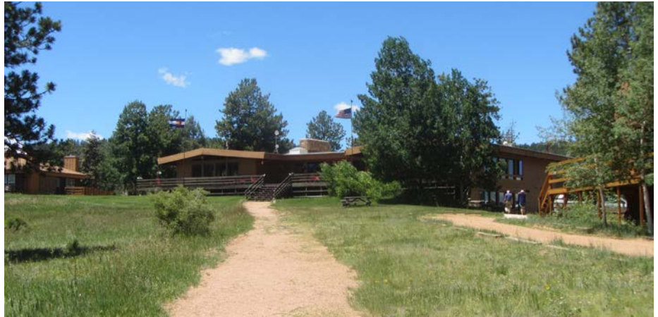
Figure 1. The main building of The Nature Place, one of the cottages is shown at the left side (Photo: Charlie Covell)
