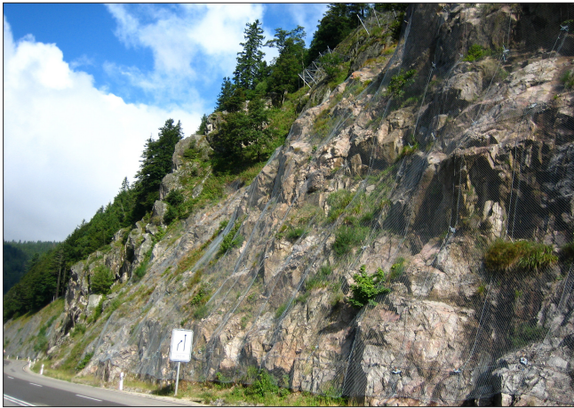
Abbildung 3. Felshang unter Steinschlag-Schutzvorhang an der B 317. - Rocky slope covered in steel wire mesh that protects the road against rock slides.
