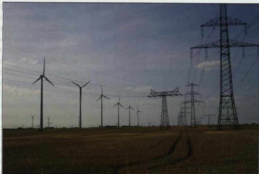
Fig. 3: High voltage pylons and wind farms near Nauen. Hobbies and Kestrels breed in Raven and Hooded Crow nests on the pylons.
