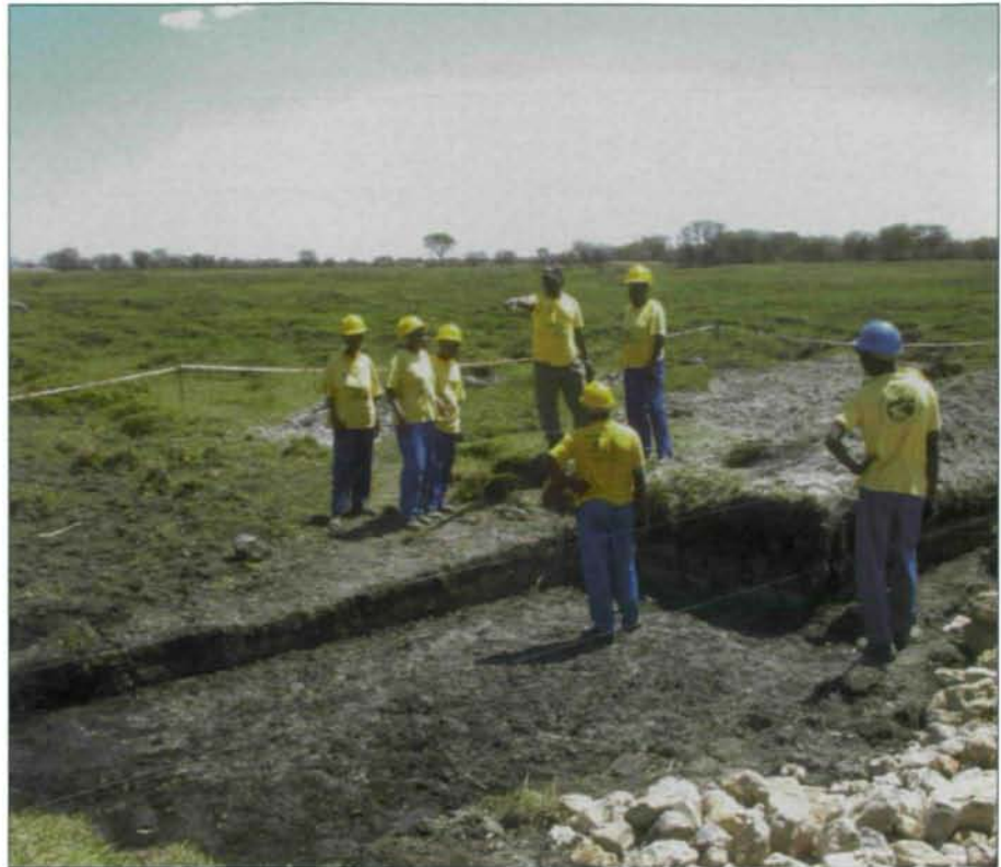
Fig. 9: A Working for Wetlands team discussing the construction of a gabion erosion control structure in a eroded gully in the Molopo peatland. Picture by Piet-Louis GRUNDLING.
