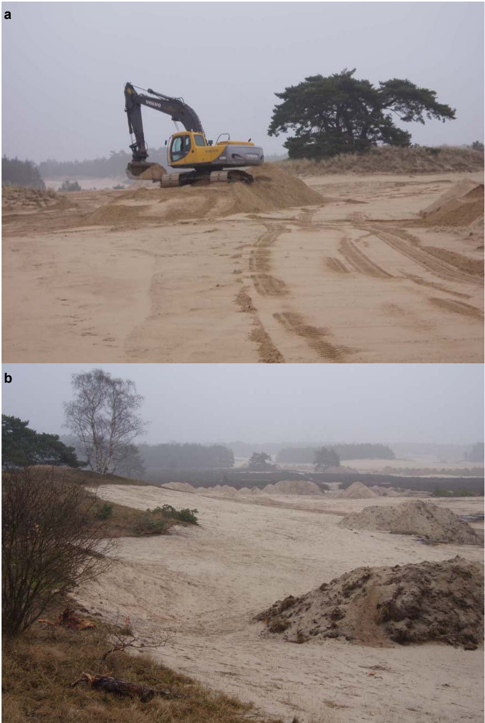
Fig. 10: Management measures carried out. a: topsoil removal at the borderline between dry heath and drift sand in 2009. b: sieving machine in action with piles of sand left after the sieving.
