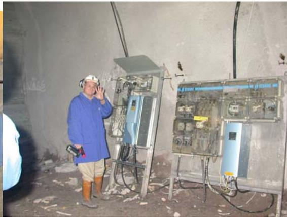
Figure 10. Fan control units with frequency inverters.
