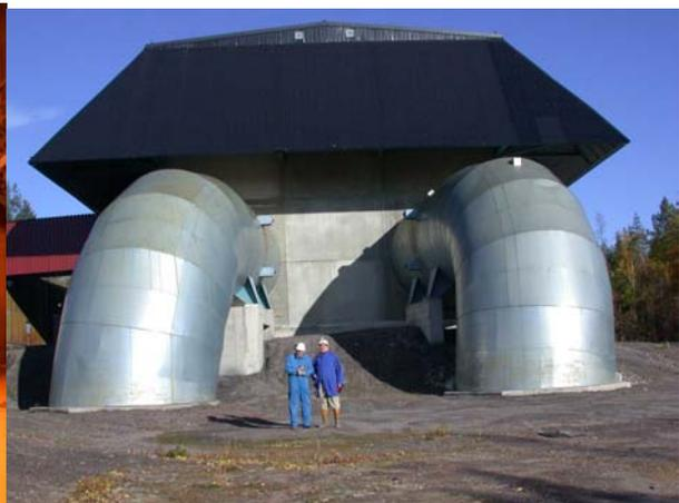
Figure 8. Air intakes for primary shafts (4.5 m diameter)
