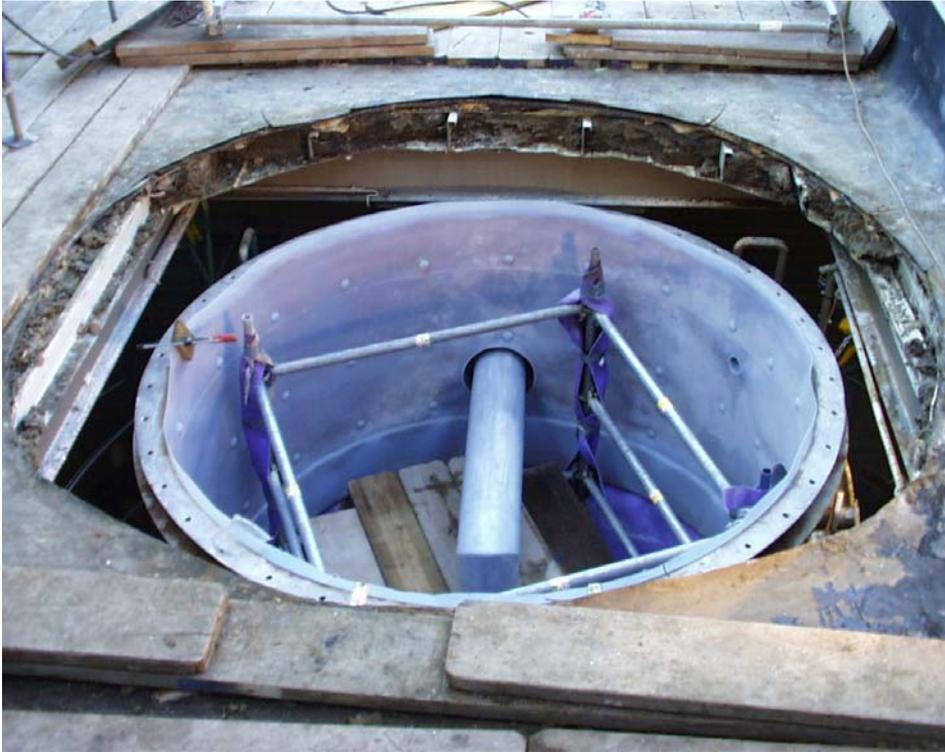
The PFA -lining is attached with a specific bolt- nut system, which is provided with welded PFA-caps on the gas loaded side.
