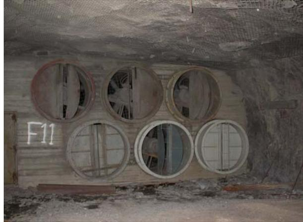
Figure 5. Fresh air ventilation wall (primary system)
