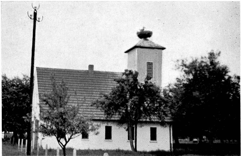
Abb. 9. Storchnest in Brockhausen.
