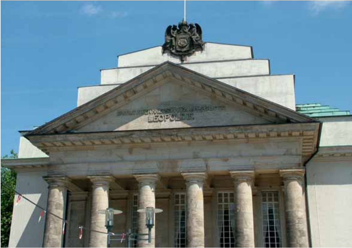
Abb. 32: Landestheater in Detmold (1914 – 1916)
